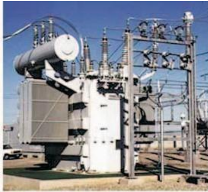
Figure 2.1 View of a Transformer
